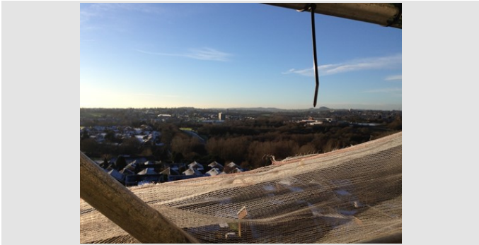
Appendix 2 Guard-rails and toe-boards:Loose
